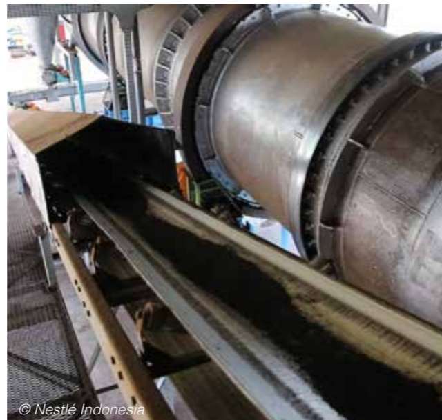
© Nestlé Indonesia The rotary dryer machine to turn leftover coffee grounds into fuel
